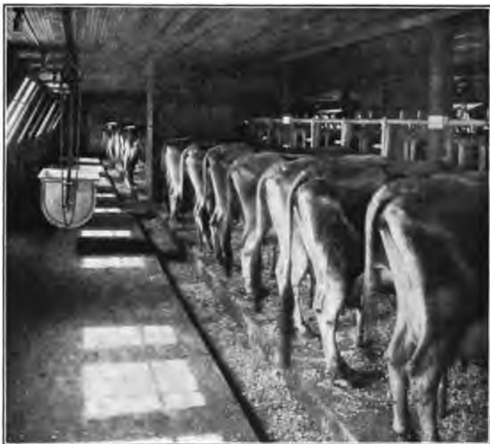
FIG. 67. — Interior view of dairy barn, showing litter-carrier, cement floor, gutter, and arrangement of windows.
